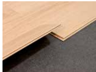
2. Press Into Place Presionar Compression
