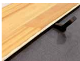
3. Press Into Place Presionar Compression
